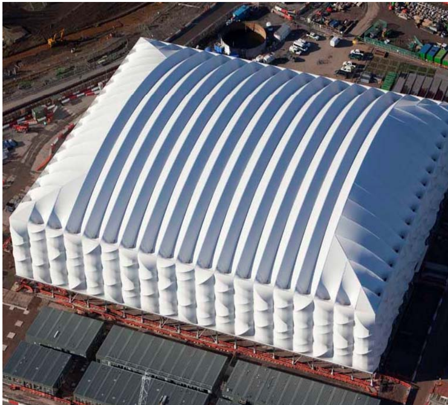
London Basketball Arena
